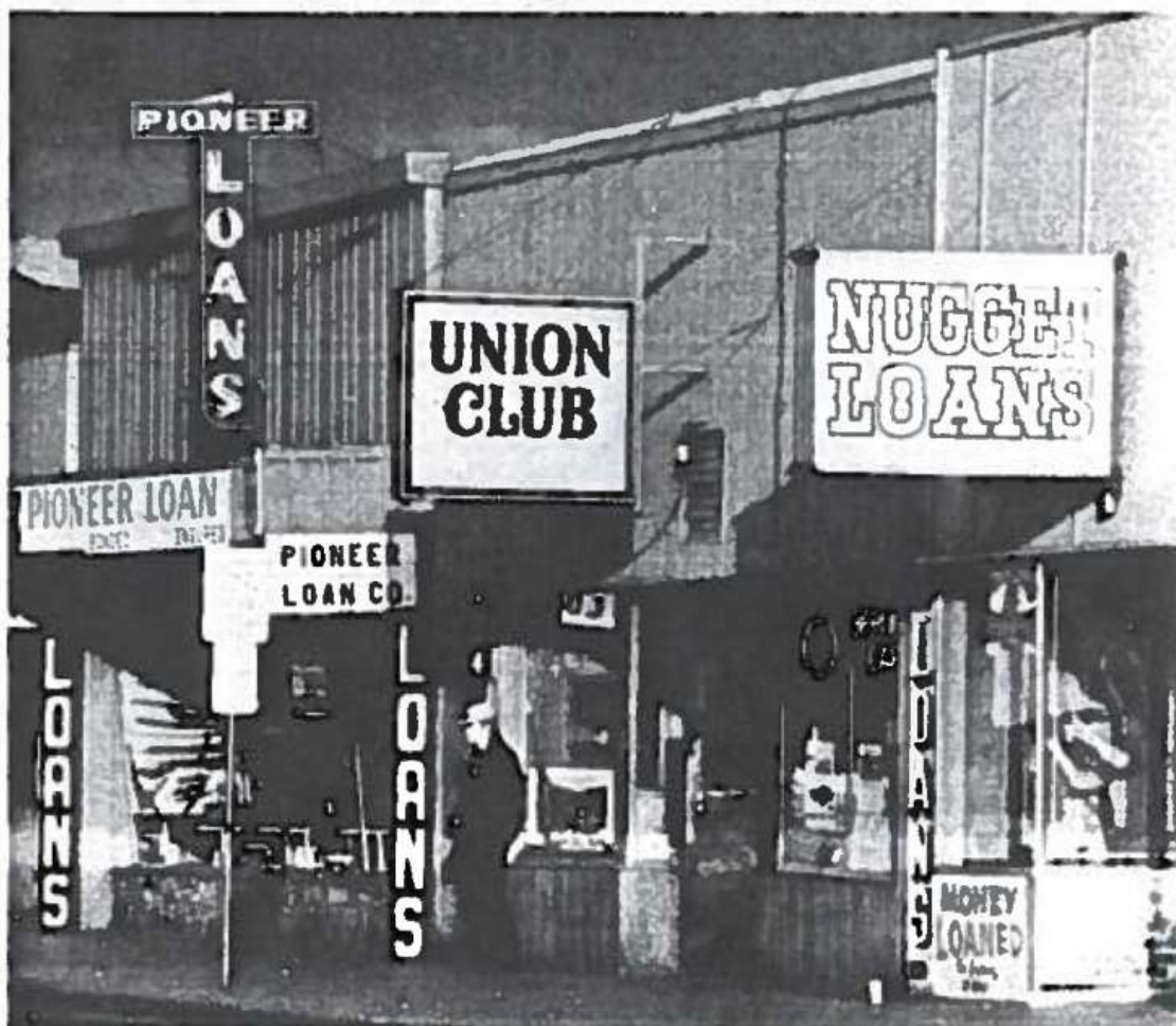
The store fronts on these two buildings have been altered over time; however, they are among the earliest buildings on Fourth Avenue.
